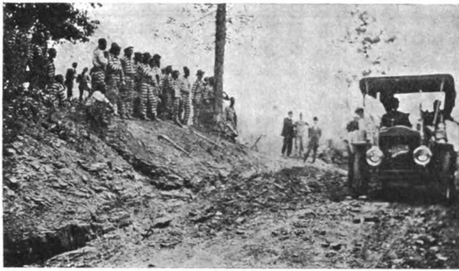
Georgia Convicts Cutting Road Through Solid Rock.
